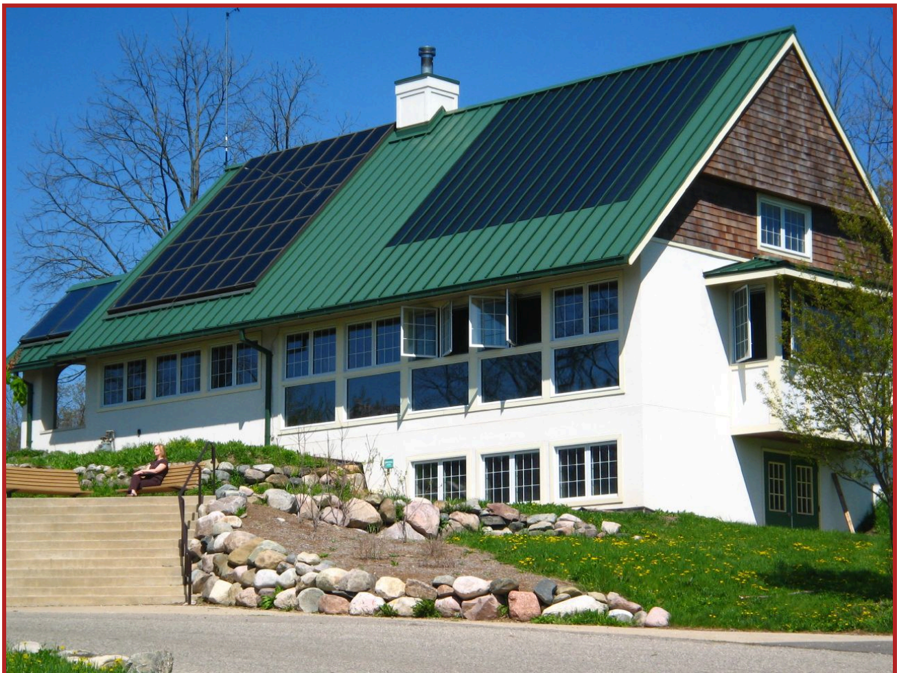
Figure 1. This roof showcases two types of solar photovoltaic systems: one standard solar panel (left) that sits on top of the roof, and the other mimicking the roof tiles (right). Courtesy of John Hritz, 2007, FlickrCommons. CC BY 2.0.
